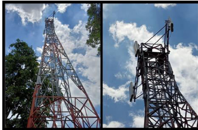
Refigure 5. TOWER STRUCTURE:
