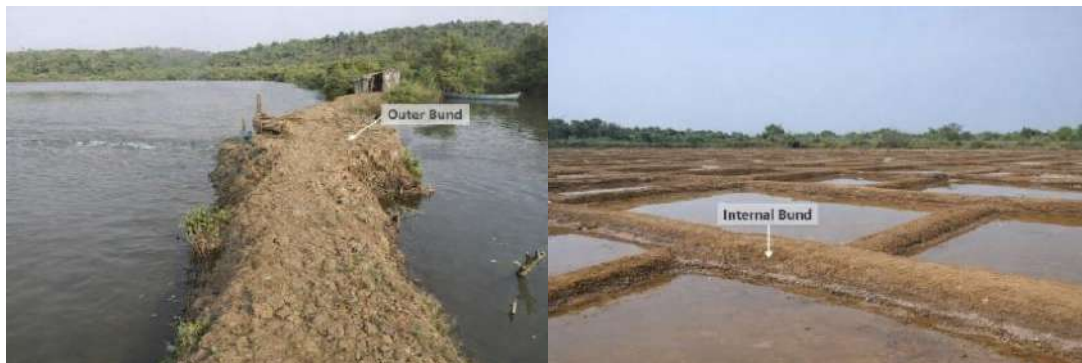
Figure 2: Bund structures of the Khazan system
